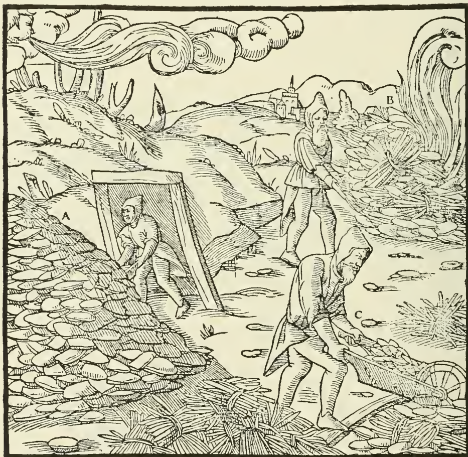
A—HEAP OF CUPRIFEROUS STONES. B—KINDLED HEAP. C—STONES BEING TAKEN TO THE BEDS OF FAGGOTS.
